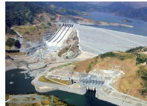
Water Storage & Hydro Power
